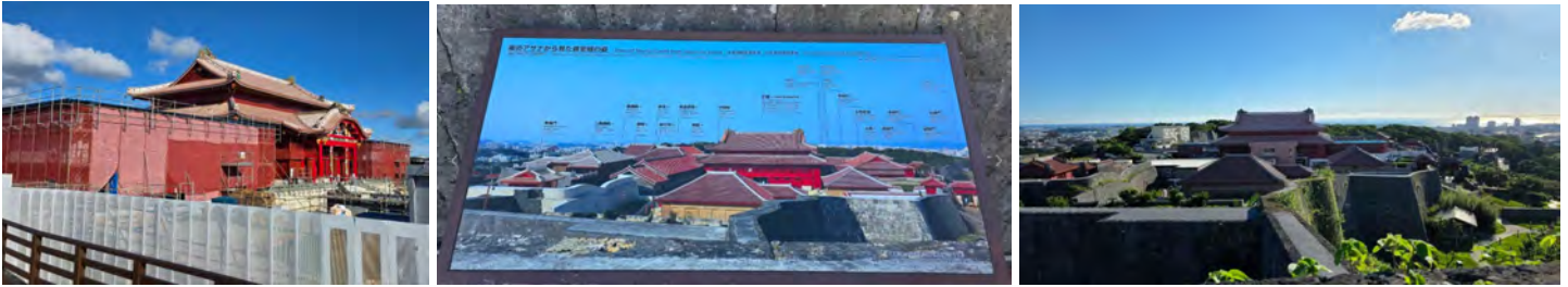
Shuri Castle: still under construction, 7 years after a devastating fire. Shuri Castle was built over 500 years ago during the Ryukyu Kingdom period.
